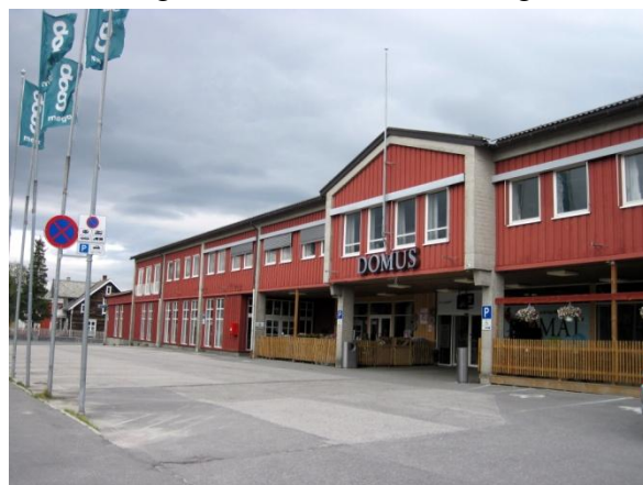
Figure 24: The mall Domus. Photo: Private
